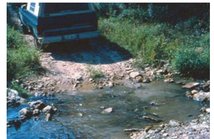
A low-water ford crossing is designed for infrequent use by vehicles.
