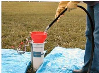
Recirculating the chlorinated water mixes the water column thoroughly and distributes the chlorine. It helps to wash down the inside sidewalls of the well casing, pump wires, and drop pipe.
