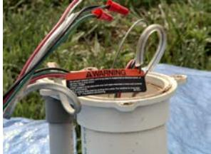
► If your well has a well cap, remove the bolts along the outside edge of the top of the well cap for newer models, or loosen the set screws on the side of the cap for older models and lift off the cap. Gently lift the wires/wire nuts out and pull to the side. Do not pull on the release cable or pull the pipe for the pitless adapter and pump. Check for damaged wires/wire nuts. Be careful not to loosen any connections.
