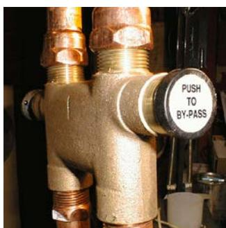
**► Bypass water softeners and other water system components, such as the dishwasher and the washing machine, that may be damaged by chlorine prior to initiating this well disinfection procedure.**
