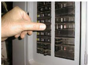
► Turn off electrical power to the pump by turning off the circuit breaker or unscrewing the fuse.
