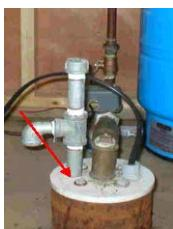
► If your well has a well seal with a threaded plug, you can remove the plug and pour the chlorine solution through the hole. If there is no threaded plug in the well seal, you should have the well disinfected by a licensed well contractor or licensed pump installer. The well seal has bolts that compress the seal. Loosening the bolts too far may cause a portion of the seal or the pump to fall into the well. **Do not remove or loosen the bolts. Do not remove the well seal.**
