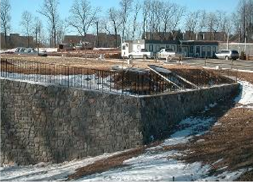
A permanent retaining wall prevents slope failure
