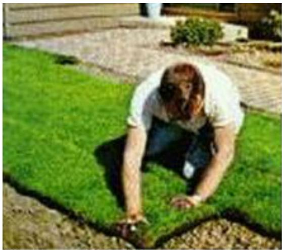
**Grass sod is laid on exposed soil to stabilize the soil and to reduce the velocity of stormwater runoff**
