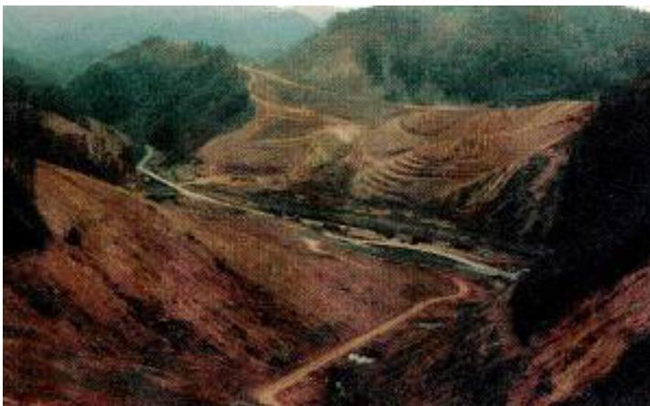
**Terraces can be incorporated into the grading plan to shorten the length of the slope and reduce the velocity of stormwater flows**
