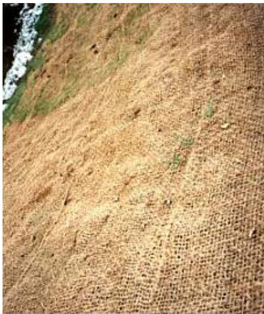
**Geotextile mats not only protect ground surfaces from wind and stormwater erosion but also allow vegetative growth (Source: Rolanka International, 2000)**
