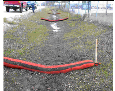
Installation of filter socks in a road ditch by Earth Corps for Indiana Department of Transportation. The filter socks will be staked through the center. Source: Filtrexx International, LLC.
