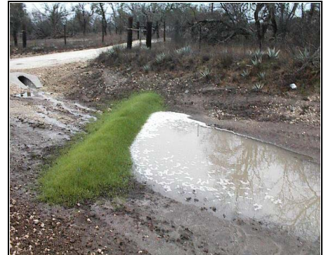
Vegetated compost filter berm. Note sediment on upstream side of berm and clear water on downstream side. Source: S. McCoy, Texas Commission on Environmental Quality.
