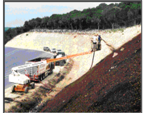
Application of a 2 inch-thick compost blanket to a 1:1 rock slope using a pneumatic blower (Austin, Texas, 2002). Source: McCoy, Texas Commission on Environmental Quality (TECQ), 2005
