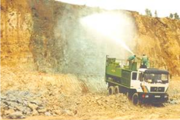
A truck applies chemical stabilizers to reduce soil erosion where vegetation can not be planted (Source: Terra Firma Industries, 1999)
