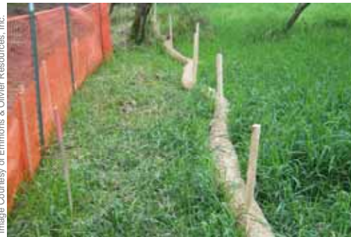
Bioroll used for perimeter control.
