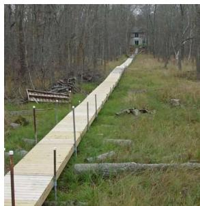
Where wetlands exist adjacent to lakeshore, boardwalks are an approved option for accessing the lake. The Minnesota Wetland Conservation Act (WCA) considers an elevated boardwalk a reasonable and prudent alternative to using fill to access the lake. The posts and pilings needed to support the boardwalk do not count as a wetland impact or 'fill.' Crow Wing County allows up to a 6 foot wide elevated boardwalk with a Shoreland Alteration Permit.
